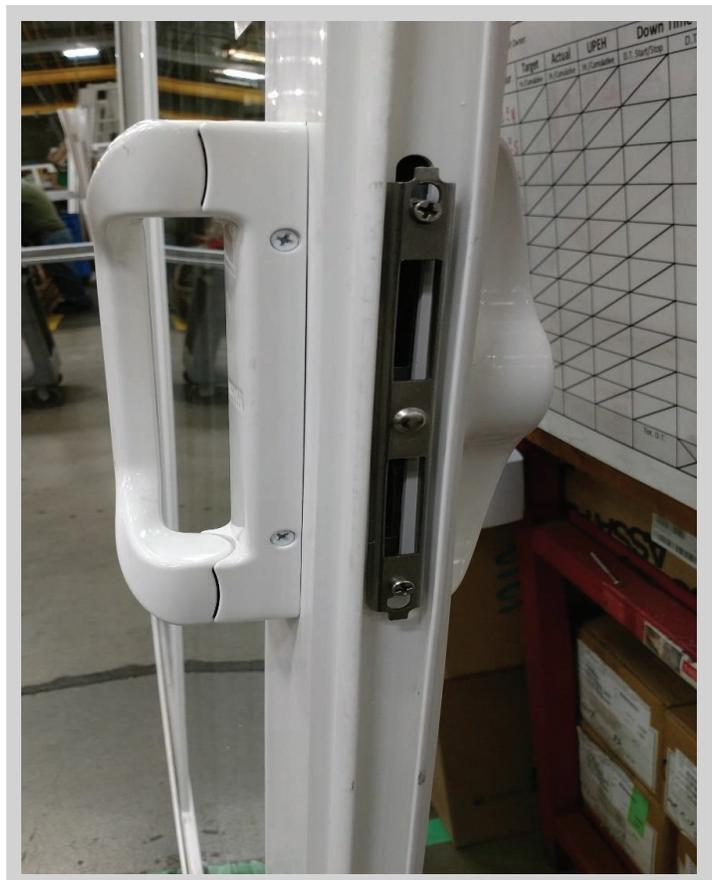
5. If active and passive panels have optional auxiliary fresh air/security bolts at top of panels, engage them as well by lifting latch.
