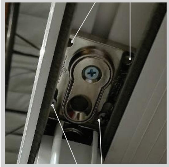
**LOOSEN SCREWS TO ADJUST STRIKE**
